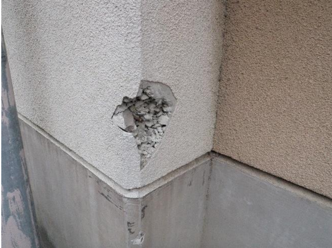
柱・外壁①
