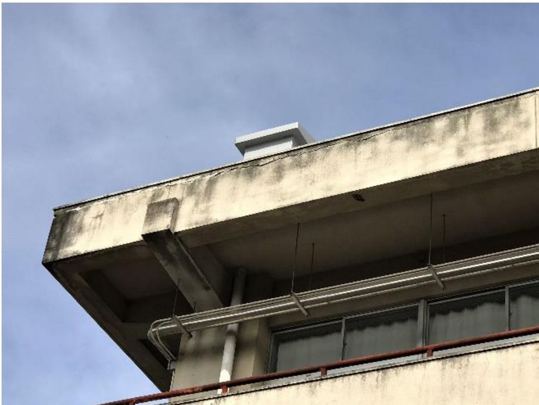
柱・外壁②
